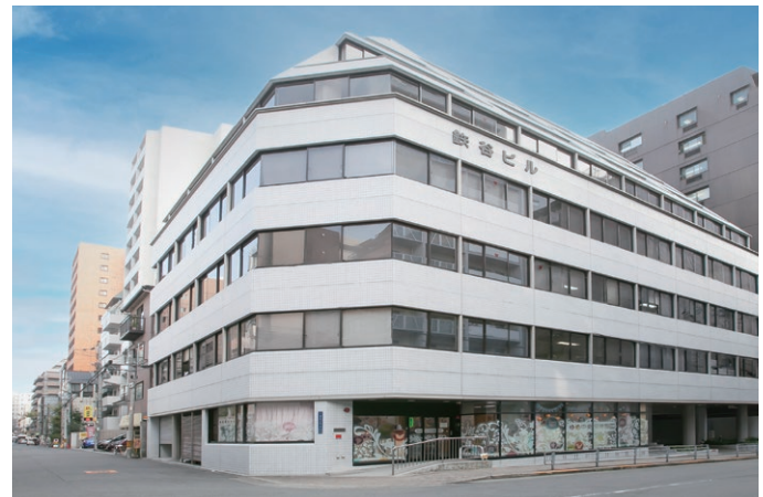
本社外観 Exterior of Headquarters
