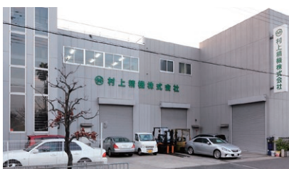
本社外観 Exterior of headquarters
